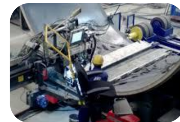
3. Cans are longitudinally welded
