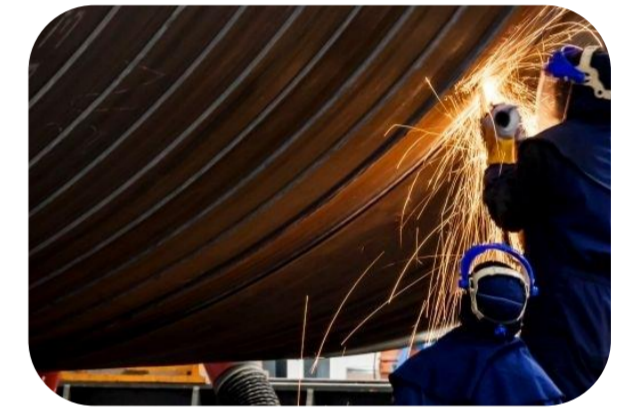
4. Cans are circumferentially welded
