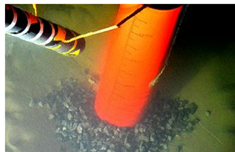
Fall pipe rock placement
