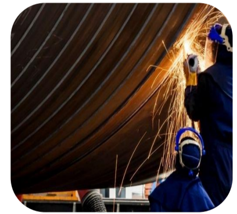
4. Cans are circumferentially welded
