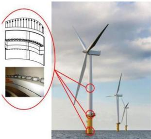
Figure 1: Showing the location of bolted connections in the offshore wind turbine.[1]
